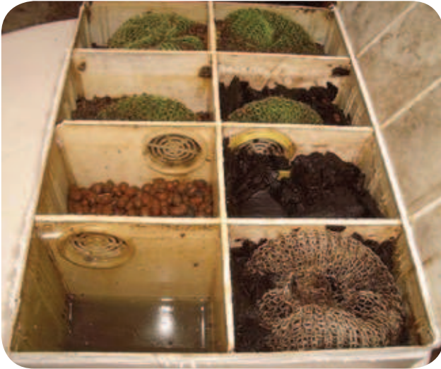
The inside of a used amalgam separator.
